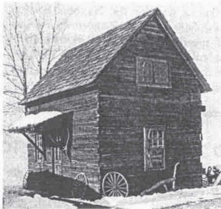
Famous "Wanship House" now at Pioneer Village dates from 1880, is of rough sawed logs and boasts two stories, but only two rooms—"upstairs, and downstairs." The outside surface of the logs has accumulated the mysterious "desert varnish" from weathering the winds, sun and rains of almost eighty years. It has been carefully restored and the interior furnished in simplicity with home accouterments of the era.
